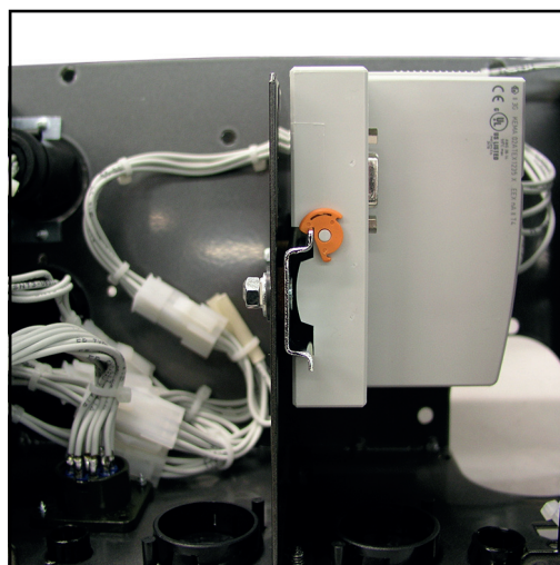
Field bus coupler fitted to insulated DIN rail
